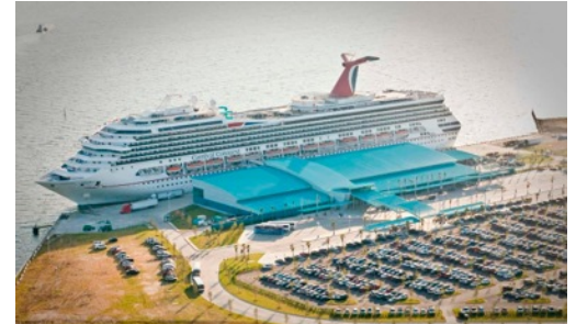
Le Port Bayport, Port of Houston Authority, Texas
